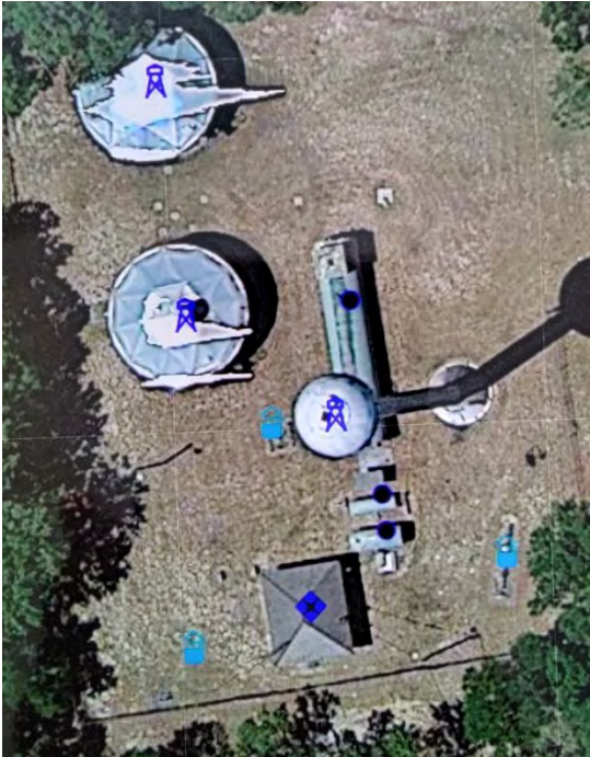
Online Water Facility
